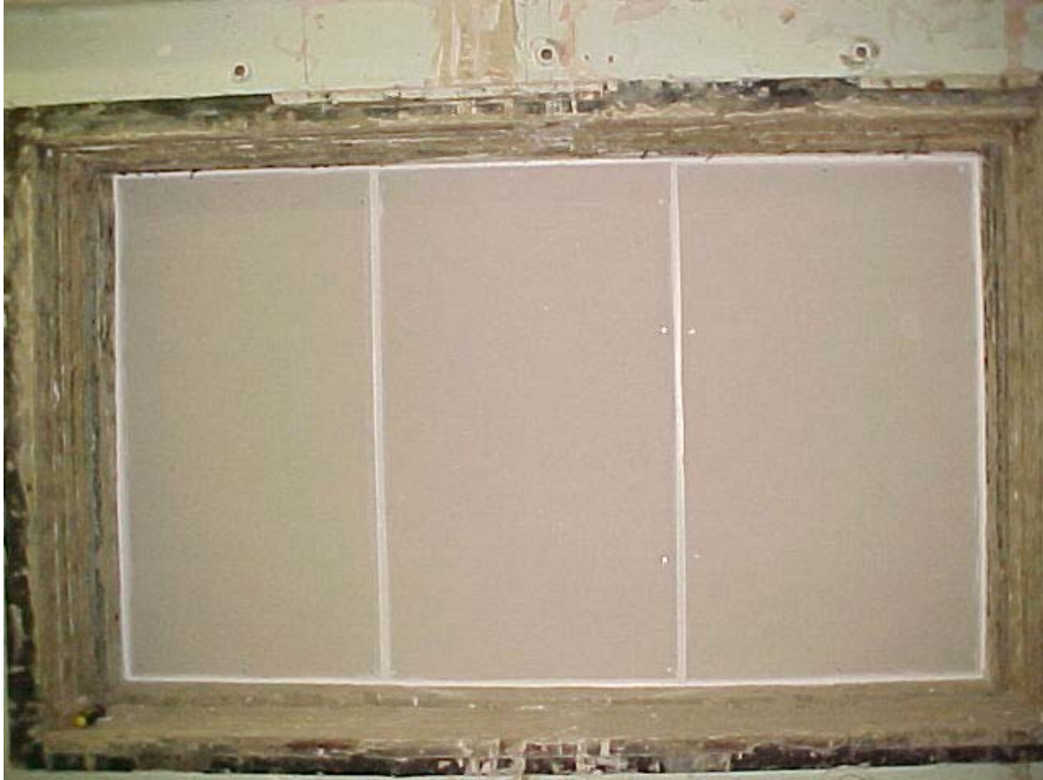
Photograph 5: Fully Sealed Partition
