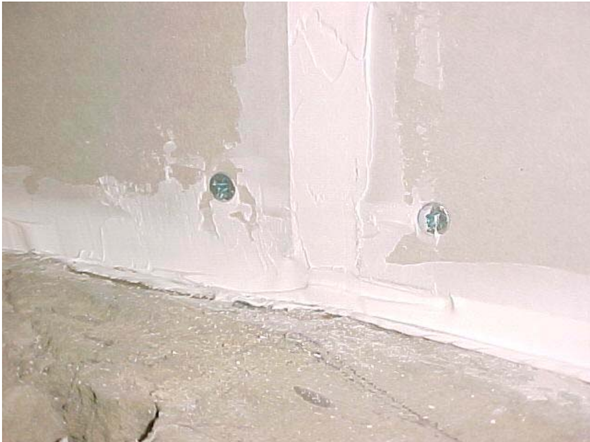
Photograph 4: Fully Sealed Partition Close-Up
